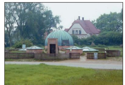
Replica of Tycho Brahe's Stjerneborg observatory on the island of Hven. The facility was placed below ground to minimize mechanical vibrations of the equipment. Motion analysis equipment has often been placed in the basement of buildings for the same reason. Observations were made through an aiming apparatus that relied on the naked eye for sighting and for reading the angular measurements. The methods were crude but the accuracy turned out to be sufficient for Kepler's needs.
